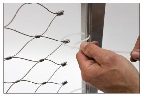
Install vertical rope clamps at one net side (vertical clamps are not absolutely necessary)! Use cable ties to install the net at end post round rod.
