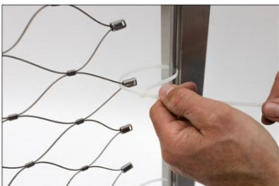
Install vertical rope clamps at one net side (vertical clamps are not absolutely necessary)!
